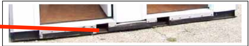
Fig. 2 - Tine Ports (Steel Frame)
